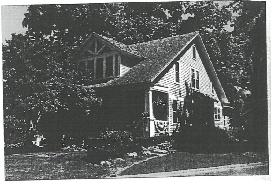
Though this New York house is clad in horizontal siding and does not show the fanciful, exposed rafter tails or pseudo-structural eave bracket associated with California, its basic form and detailing qualify it as a bungalow.
