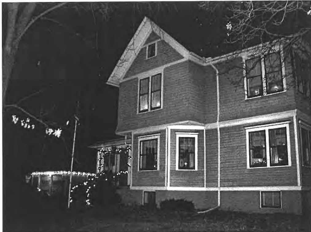
Photo of house from corner of Highland and N. Commonwealth
