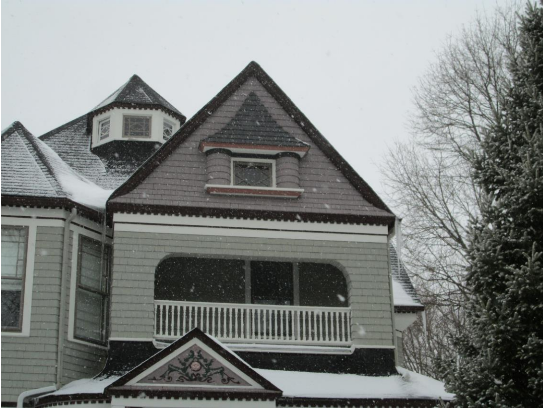
East balcony, gable and dormer
