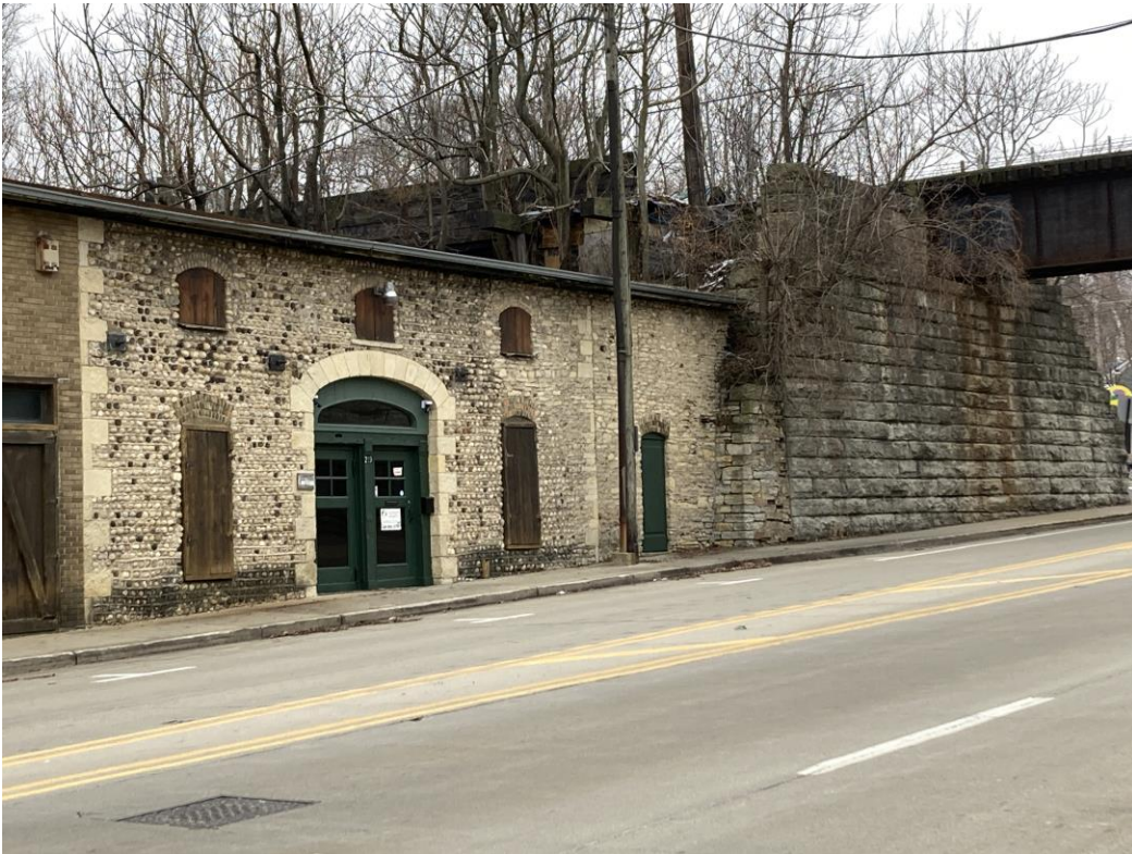
North elevation with railroad trestle
